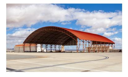
The **COVERED CORROSION AIRCRAFT WASH FACILITY** accommodates aircraft as large as a C-5 in size and is lighted for 24-hour operation. Available equipment includes a soap foamer and two high-pressure, hot-water wash units.
